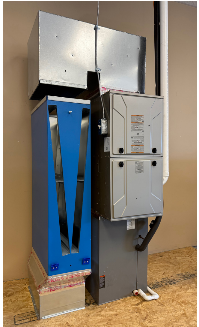
Figure 3G. Install filter cabinet.
