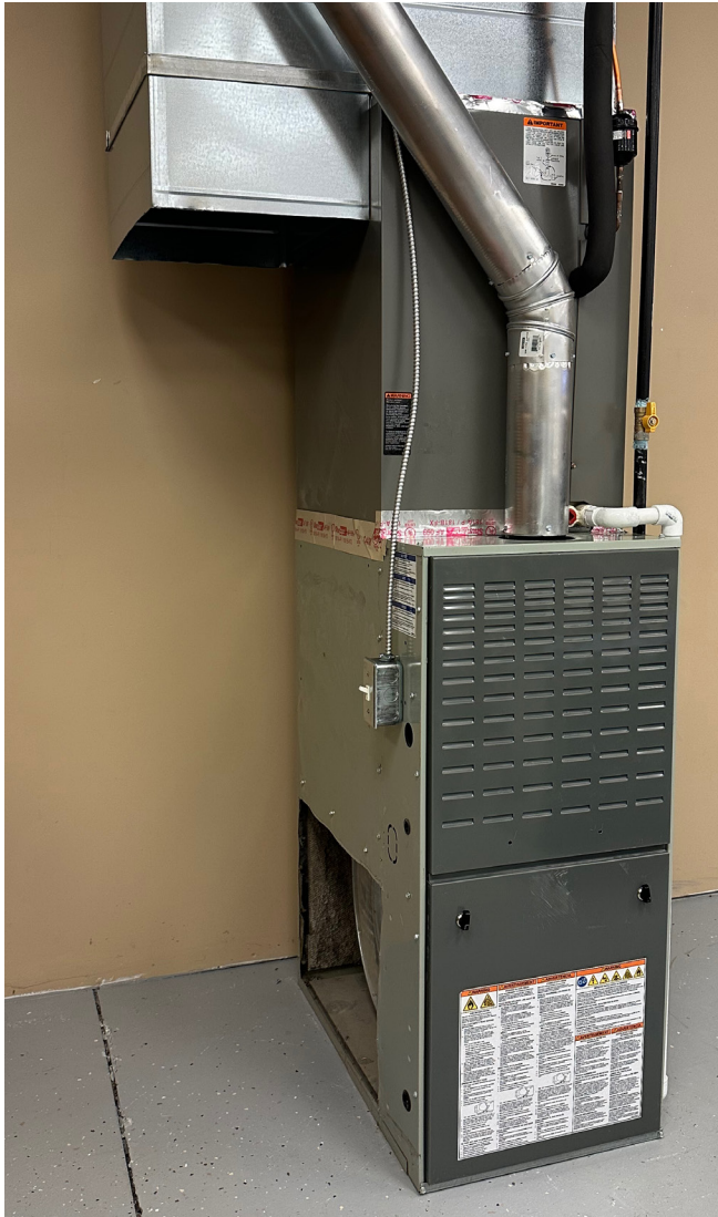
Figure 1C. Remove return air duct.
