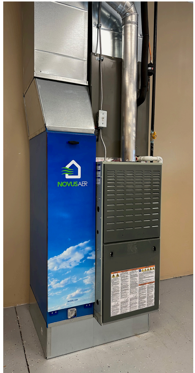
Figure 6N. Install cabinet door.
