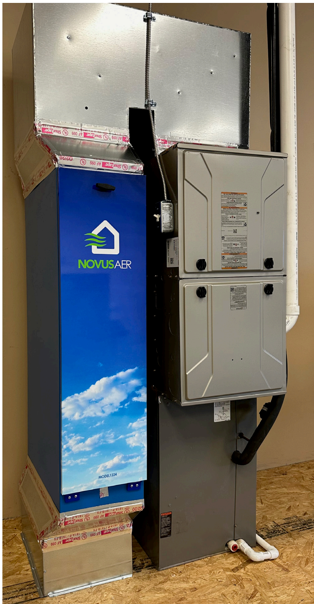
Figure 3K. Install filter cabinet door.
