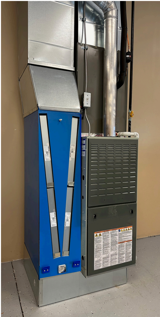
Figure 6M. Install air filters.
