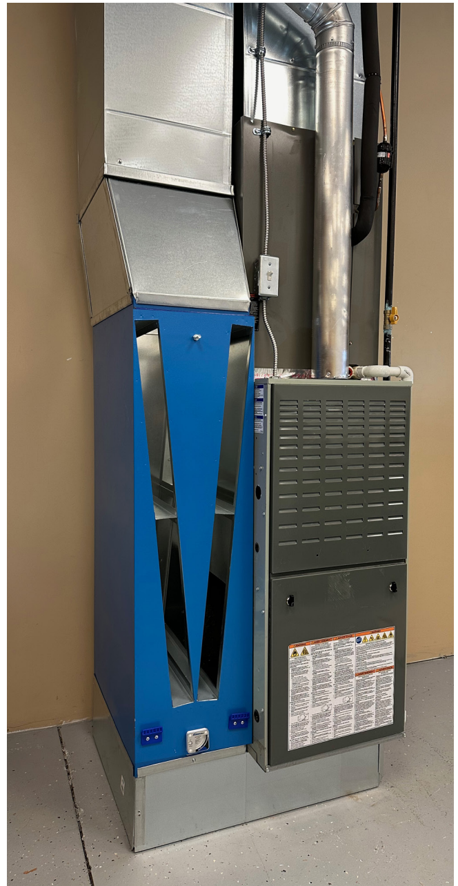
Figure 6L. Install upper transition.
