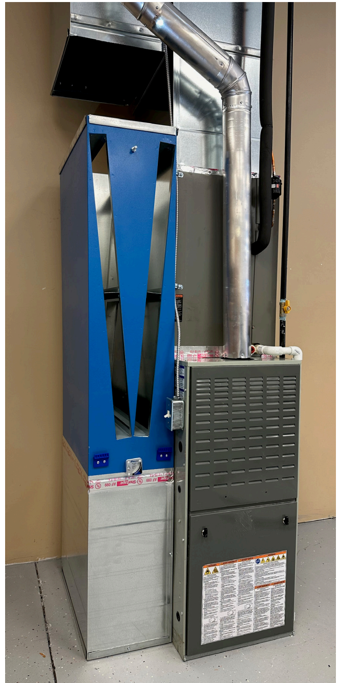
Figure 2L. Install cabinet assembly on furnace/air handler.
