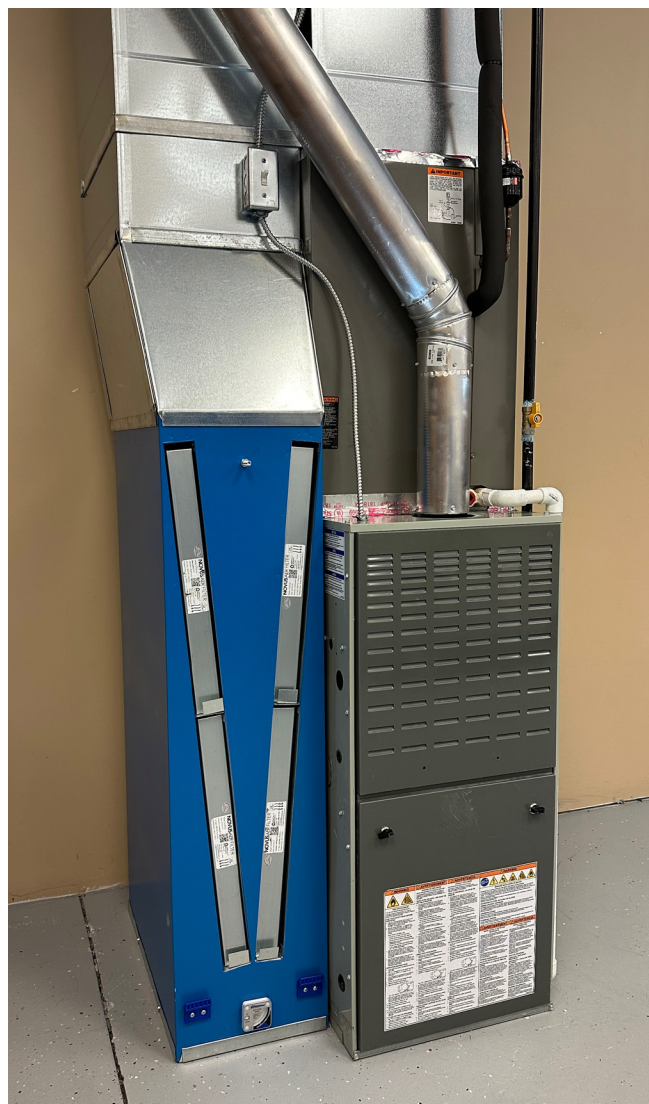
Figure 1K. Install the filters.
