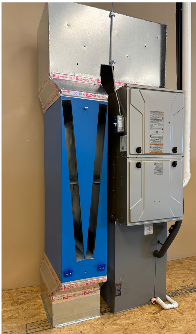
Figure 3H. Install and seal upper transition duct.
