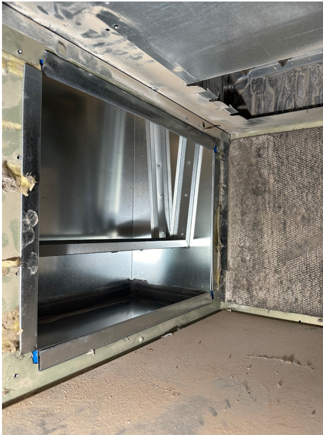
Figure 1H2. Seal the connection with s-cleats.
