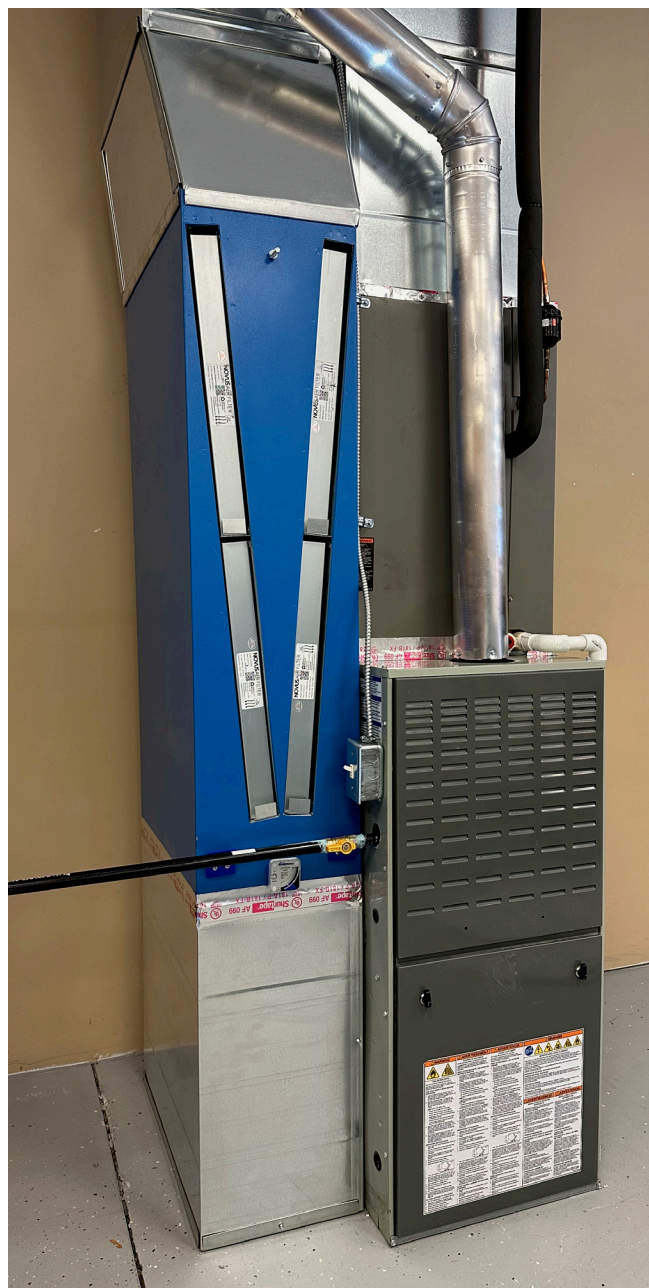
Figure 2N. Install air filters.
