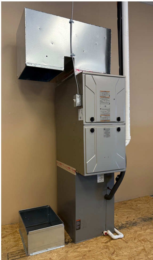
Figure 3C. Remove a section of return air duct.
