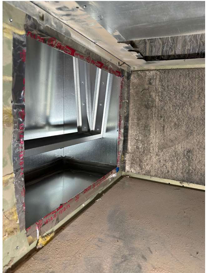
Figure 1H3. Seal the connection with tape.
