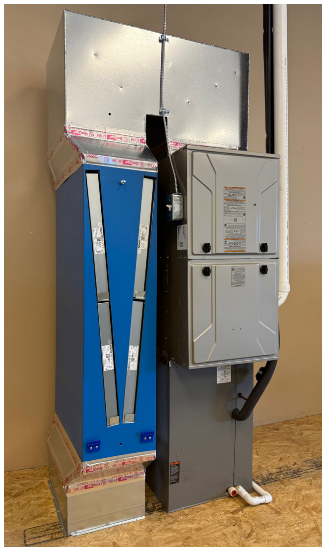
Figure 3J. Install the air filters
