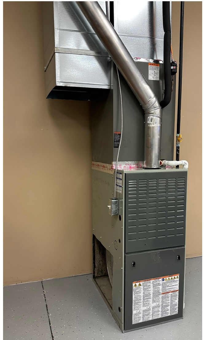
Figure 2C. Remove return air duct.
