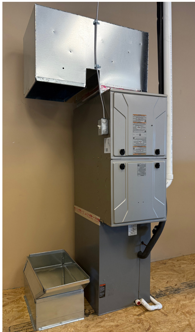
Figure 3D. Install the transition
