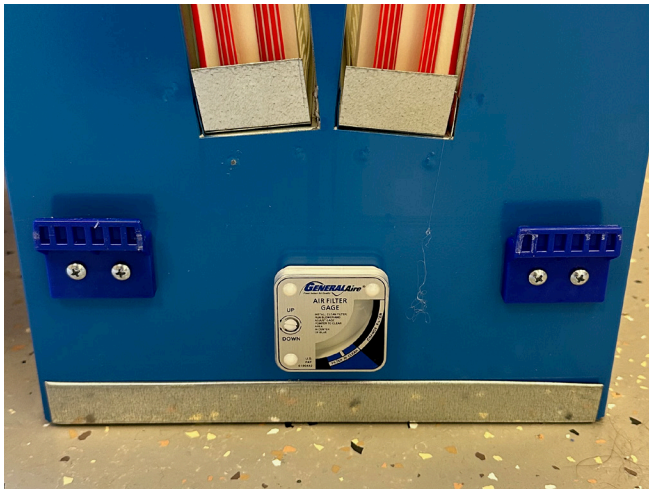
Figure 1G3. Install the air filter gauge.
