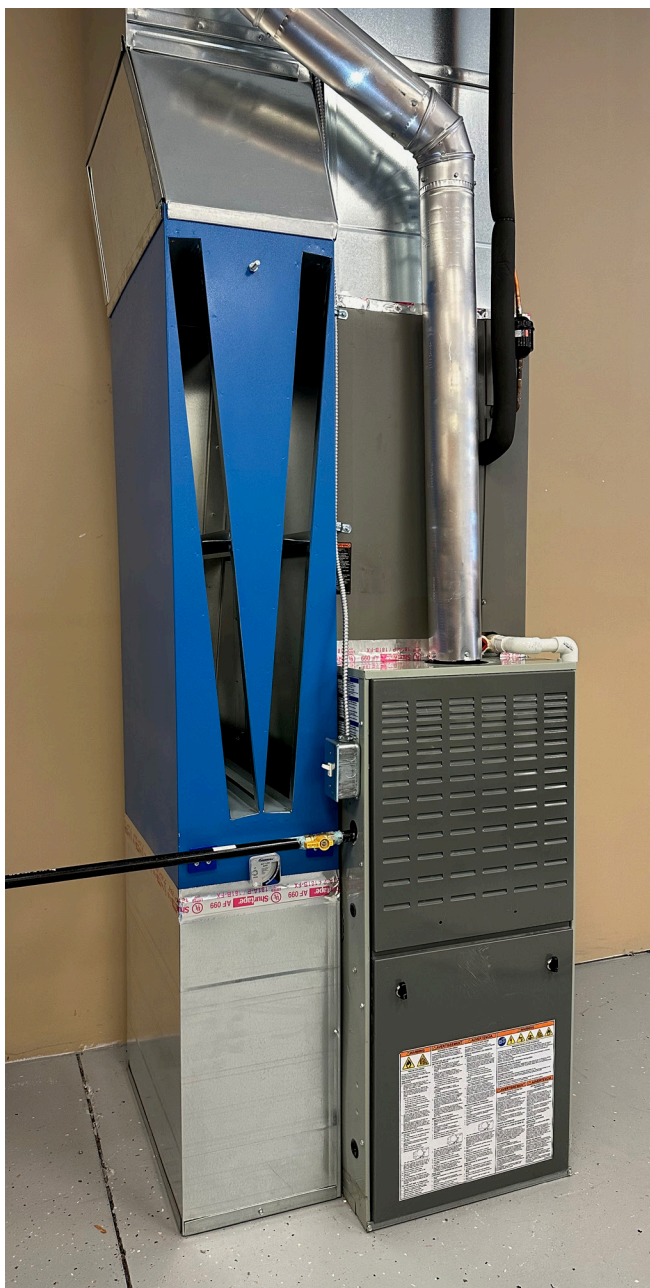
Figure 2 M. Install and seal duct transition.
