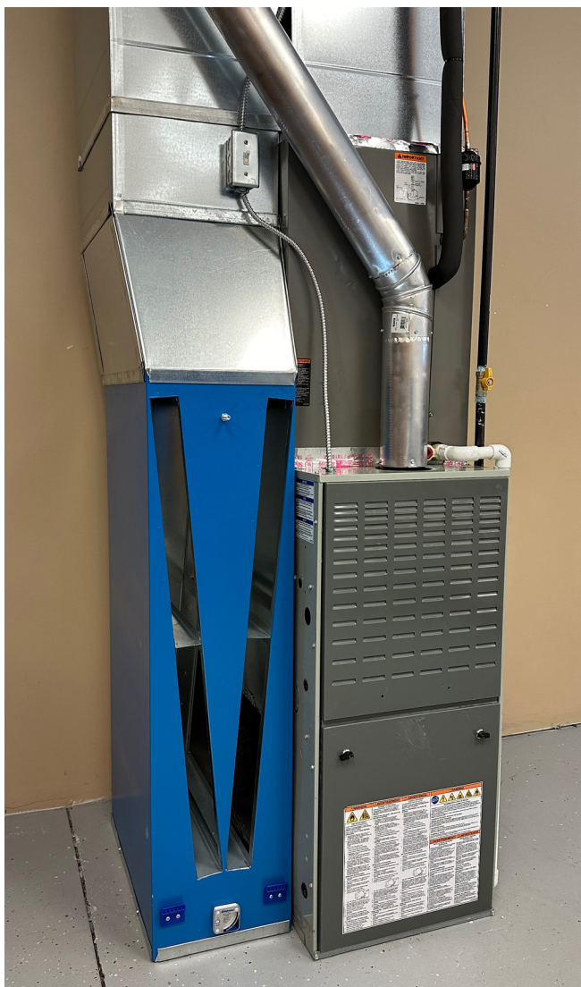
Figure 1J. Install the transition
