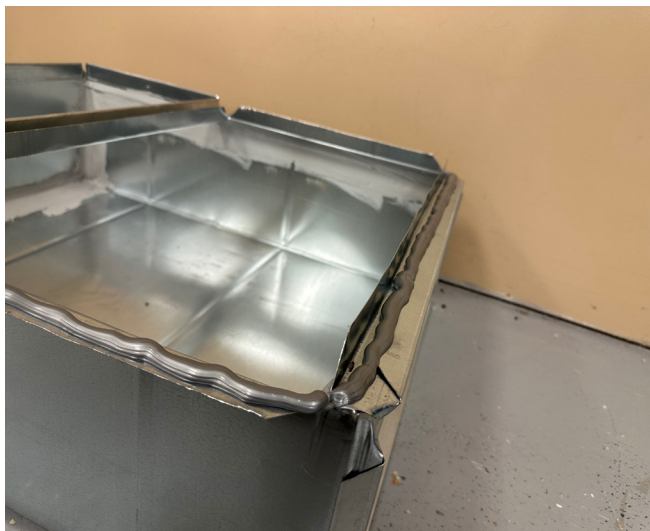
Figure 6D2. Put sealant on connecting surfaces.
