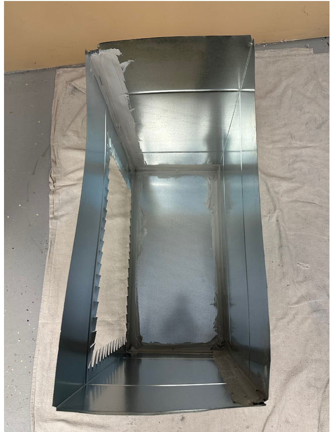
Figure 2F. Seal the extension box.
