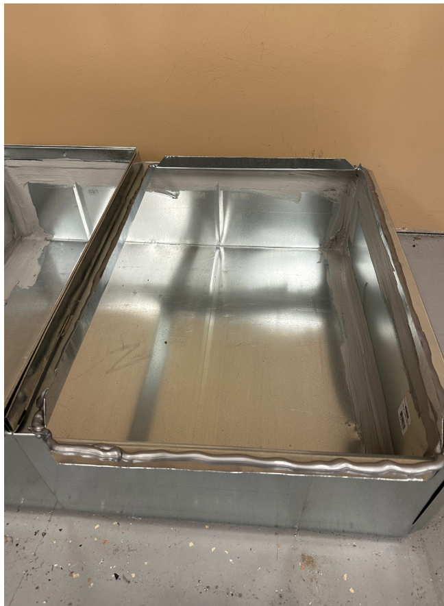
Figure 6D1. Put sealant on connecting surfaces.
