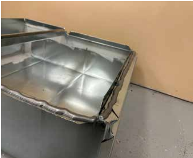
Figure 6D2. Put sealant on connecting surfaces.
