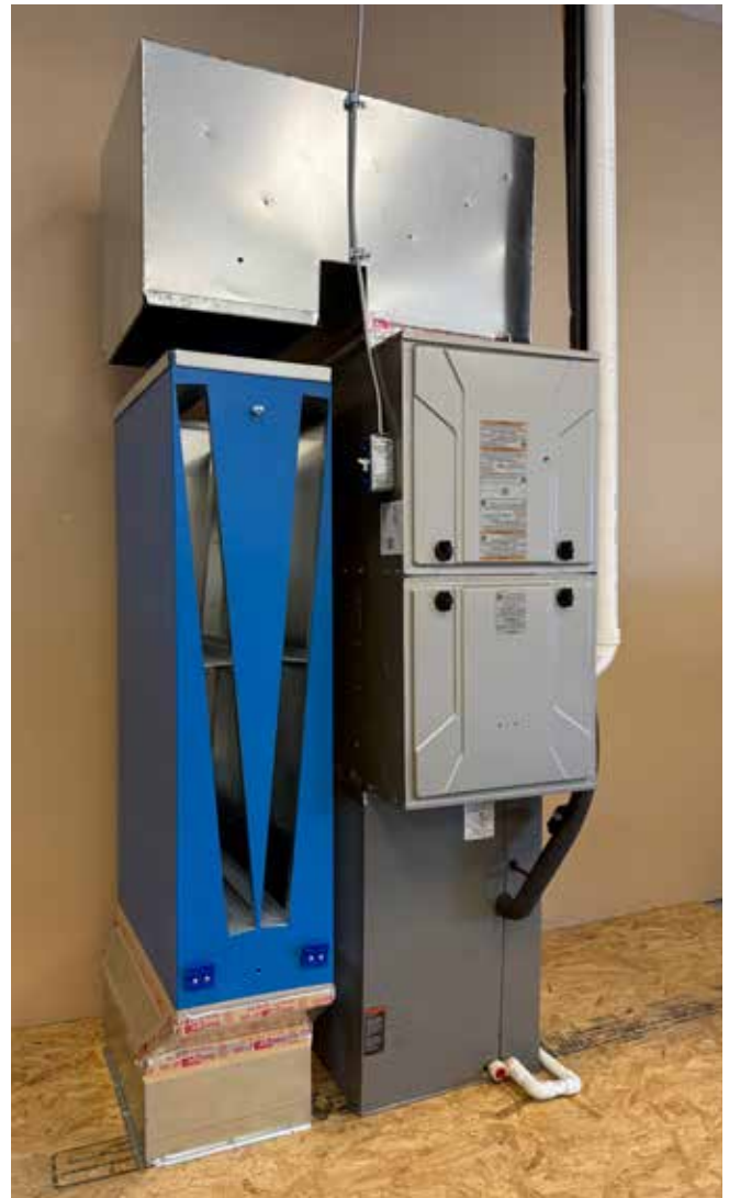
Figure 3G. Install filter cabinet.
