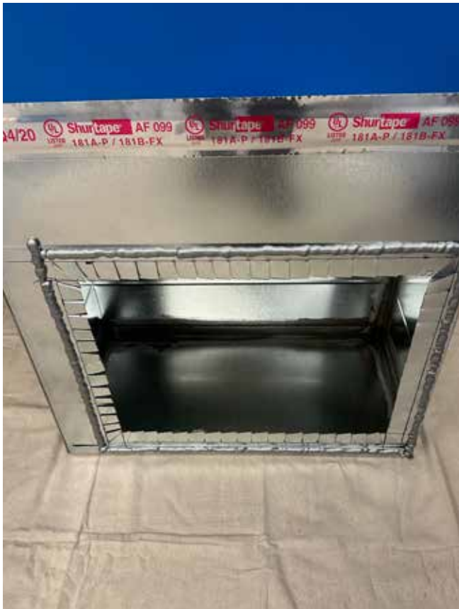
Figure 2K. Install and seal extension box.
