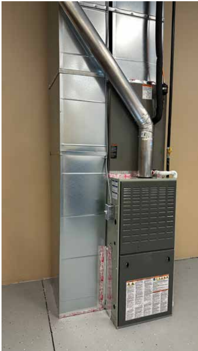
Figure 6B Typical Intallation
