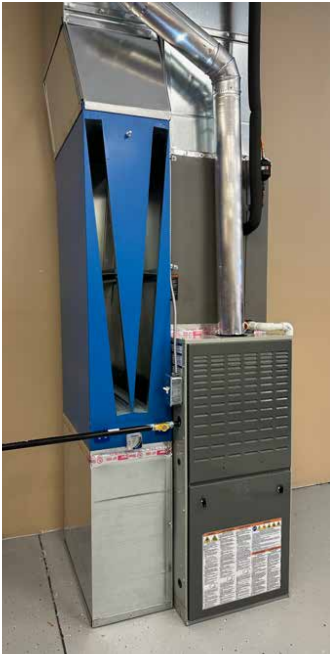
Figure 2 M. Install and seal duct transition.
