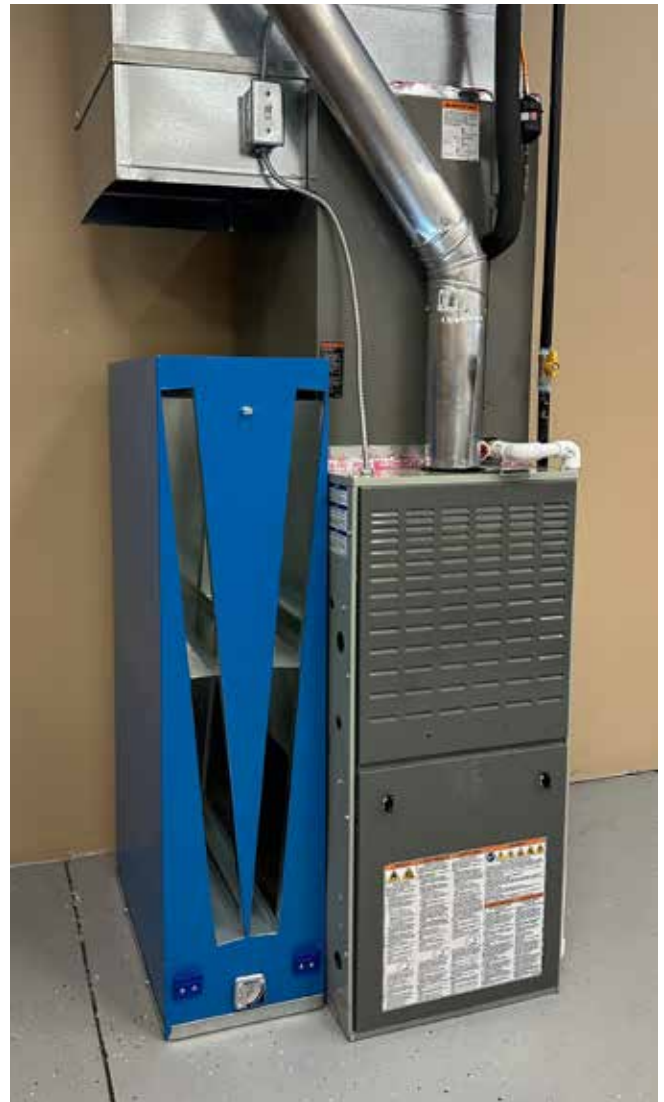
Figure 1H1. Install the cabinet on the furnace/air handler.
