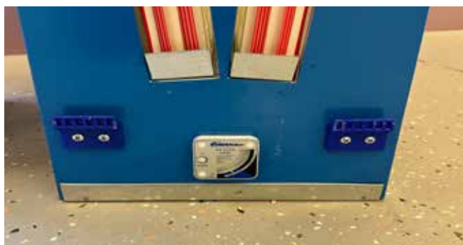
Figure 2J. Install filter gauge
