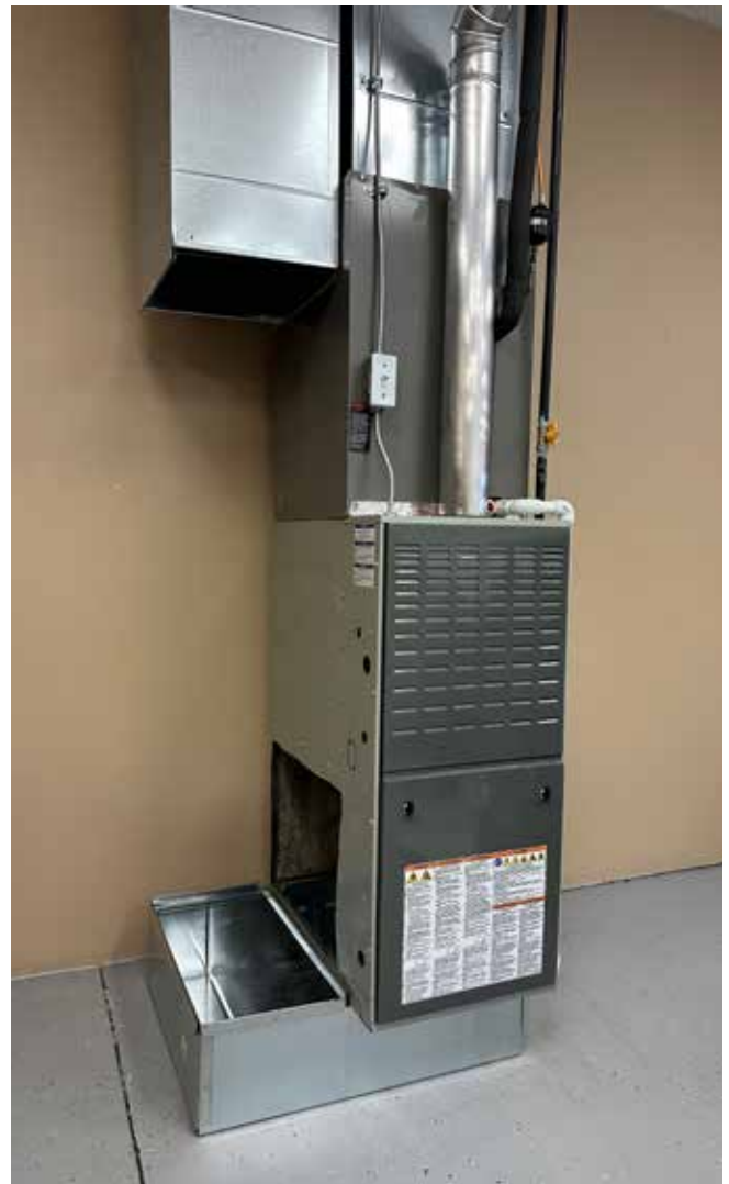
Figure 6E. Remove duct. Set the Furnace on the base.
