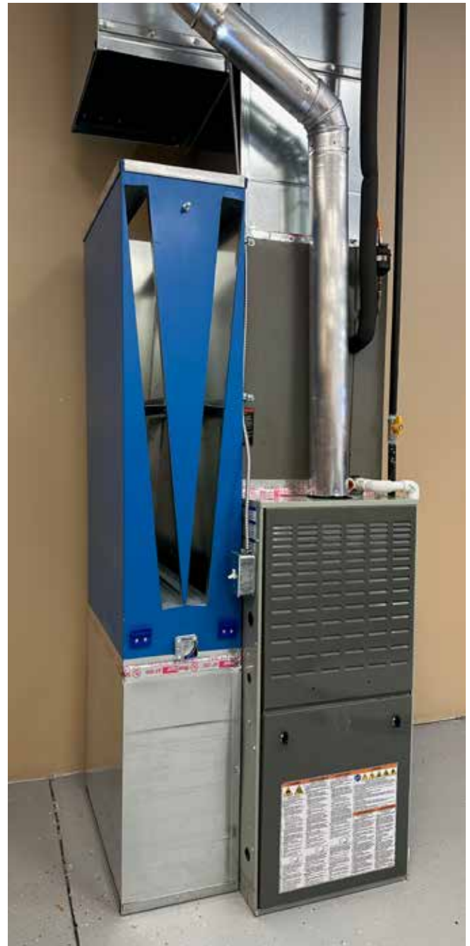
Figure 2L. Install cabinet assembly on furnace/air handler.
