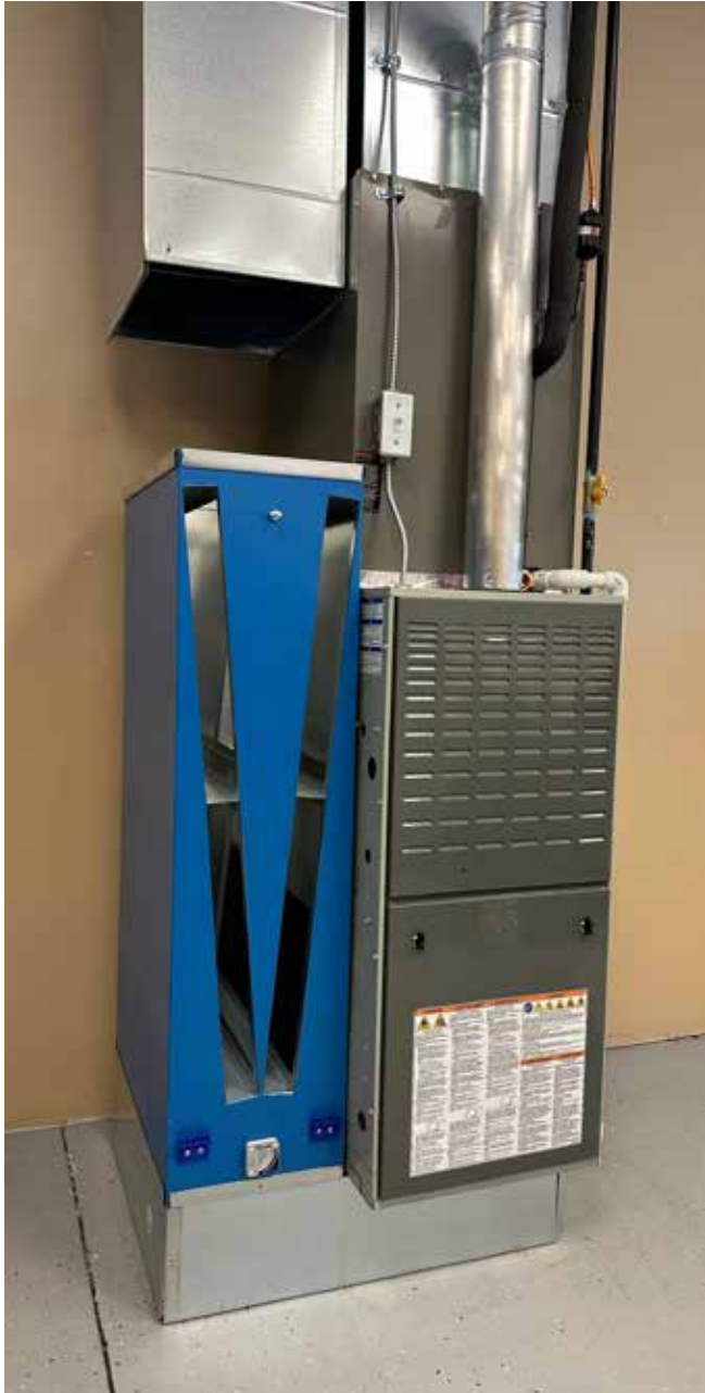
Figure 6K. Install and seal the cabinet to the base and the furnace.
