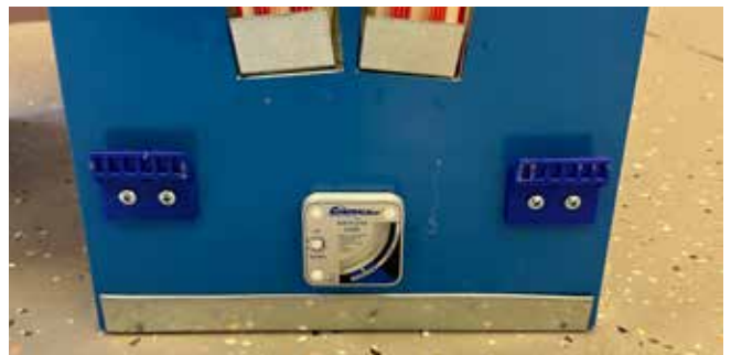
Figure 6J. Install filter gauge.
