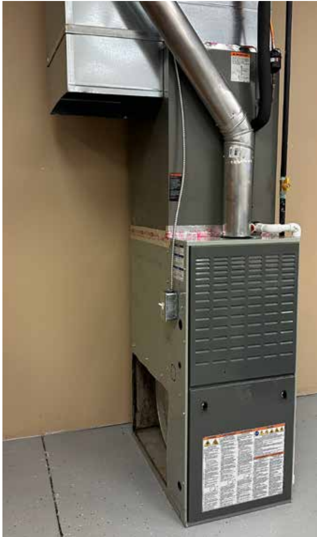
Figure 1C. Remove return air duct.
