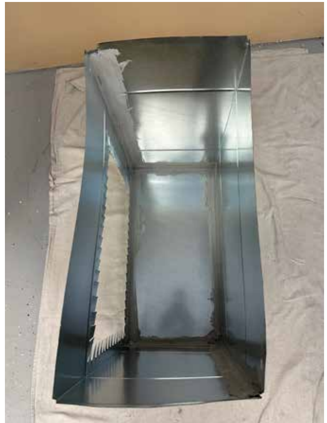
Figure 2F. Seal the extension box.
