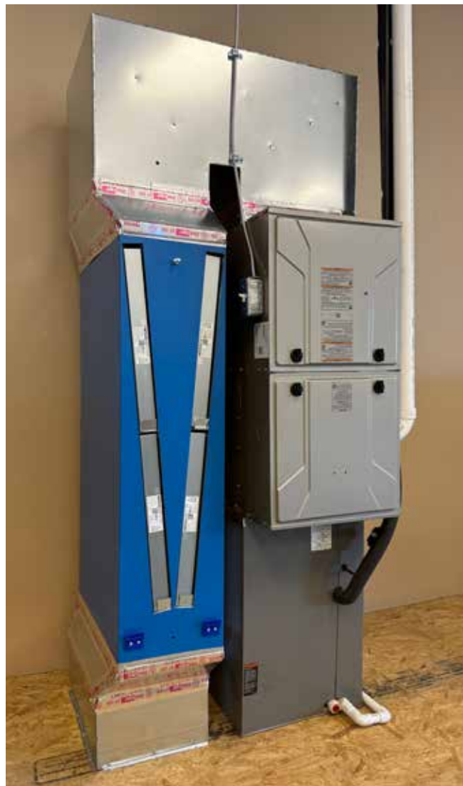
Figure 3J. Install the air filters
