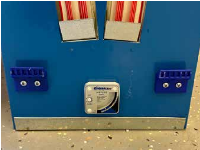
Figure 1G3. Install the air filter gauge.
