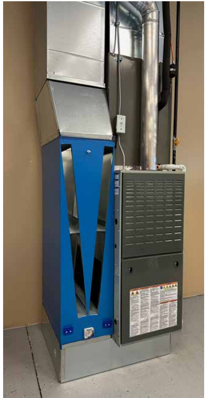
Figure 6L. Install upper transition.
