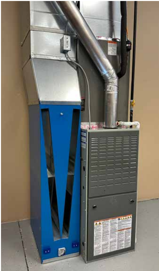
Figure 1J. Install the transition
