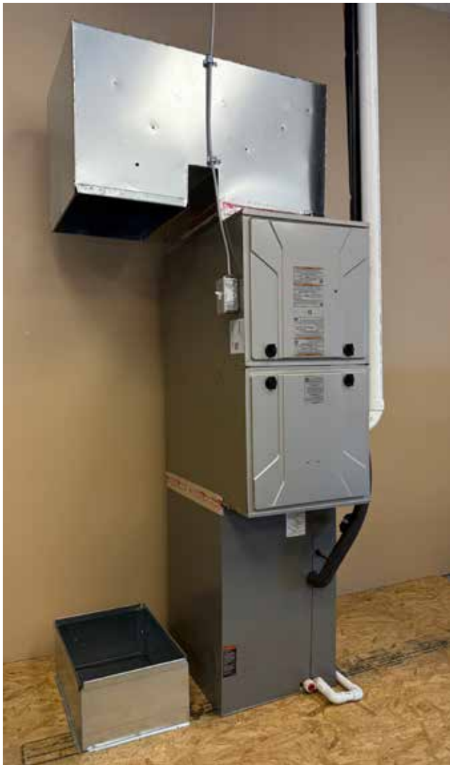
Figure 3C. Remove a section of return air duct.
