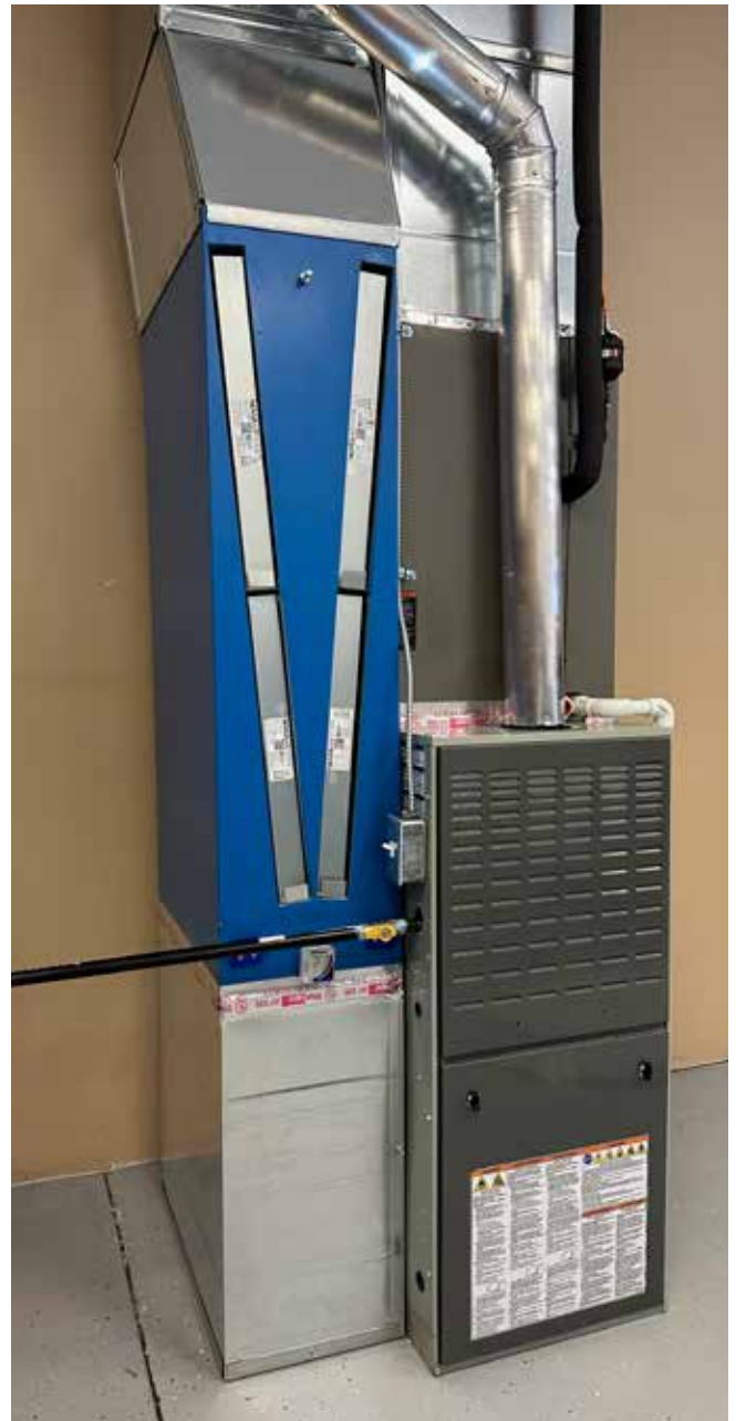
Figure 2N. Install air filters.
