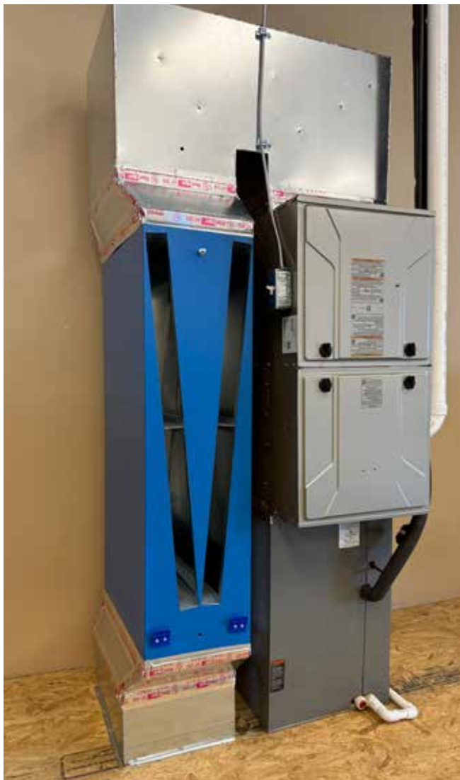
Figure 3H. Install and seal upper transition duct.
