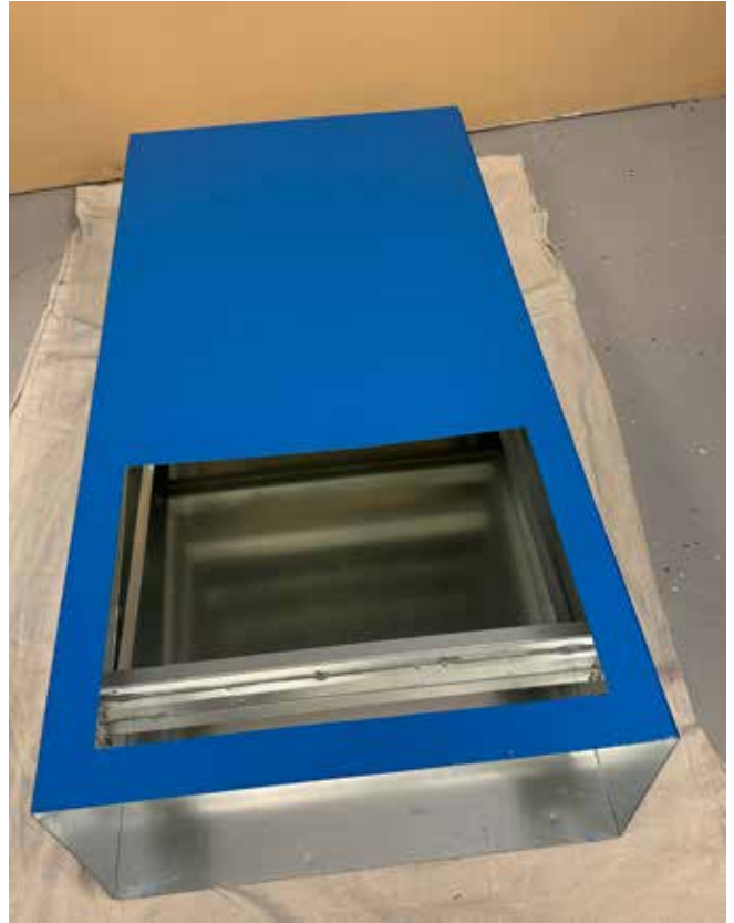
Figure 6H. Cut an opening in the side to match the furnace.
