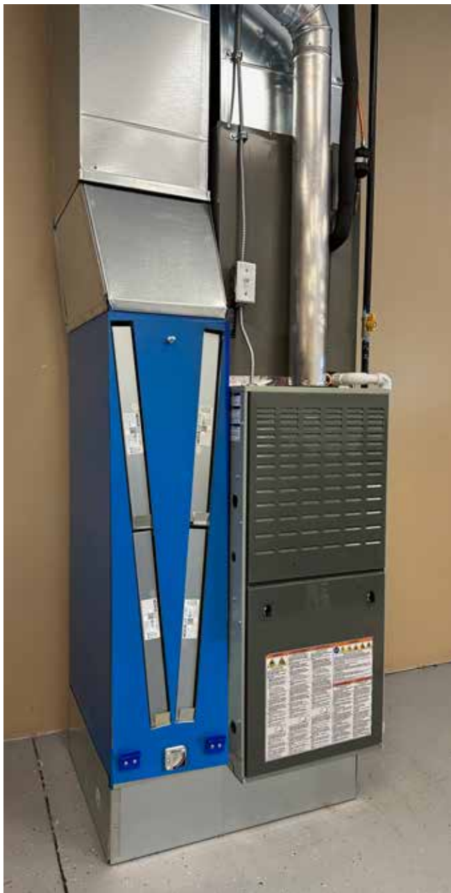
Figure 6M. Install air filters.
