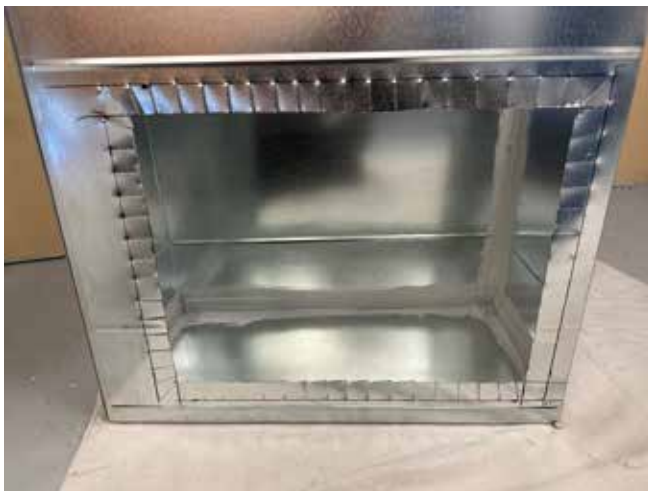
Figure 2E. Cut opening in the side of the box
