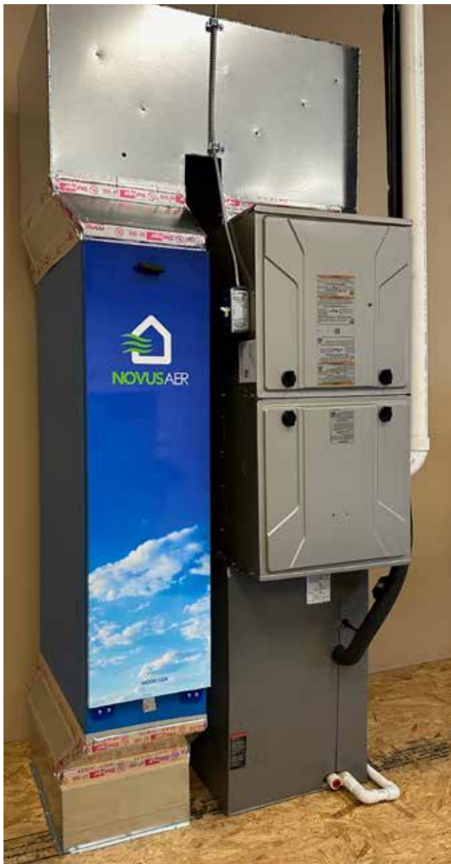
Figure 3K. Install filter cabinet door.
