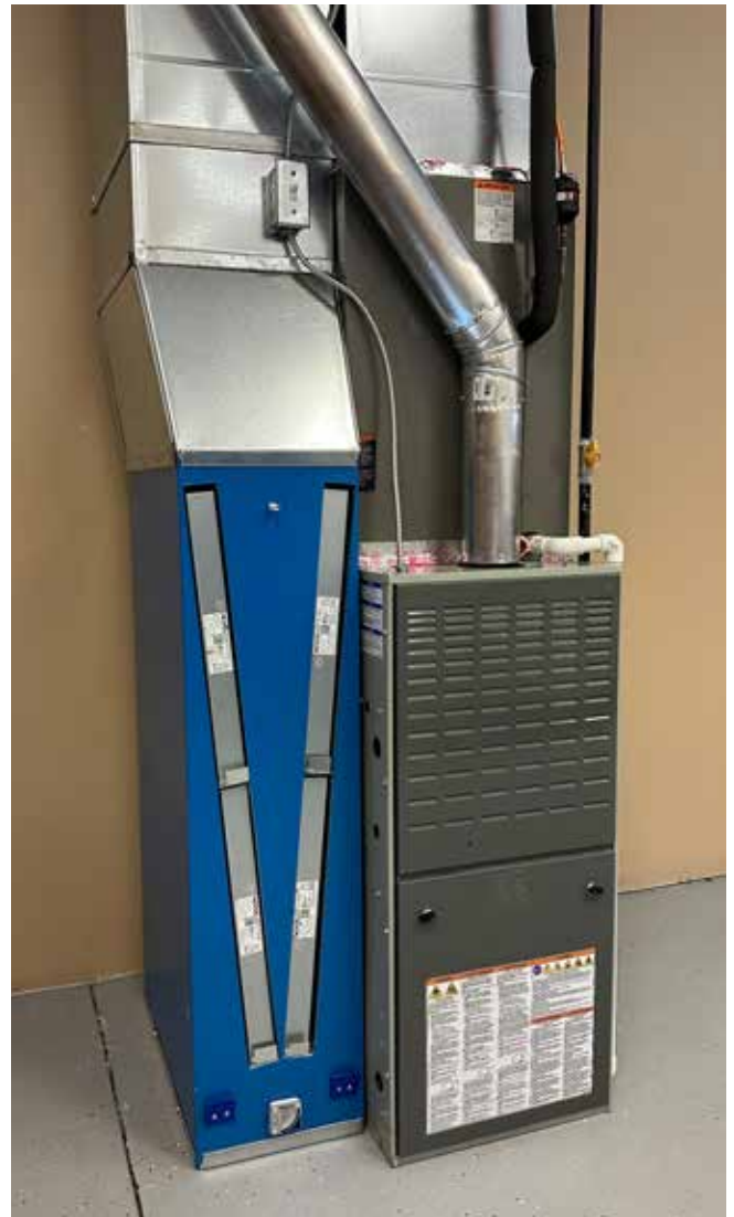
Figure 1K. Install the filters.
