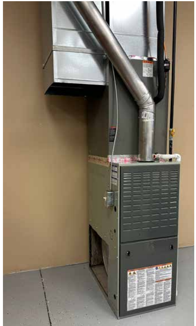
Figure 2C. Remove return air duct.
