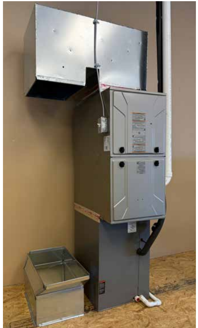
Figure 3D. Install the transition
